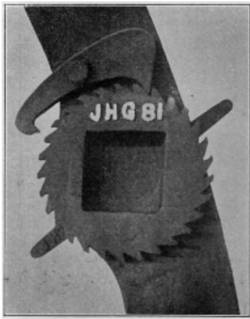
FIG. 2. A VIEW OF ONE OF THE RATCHETS IN THE GILES DYEING MACHINE
