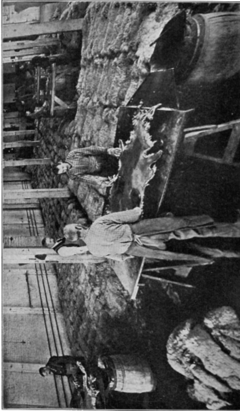
Fig. 72.—Painting Room, Applying Depilatory to Flesh Side of Pelts.
