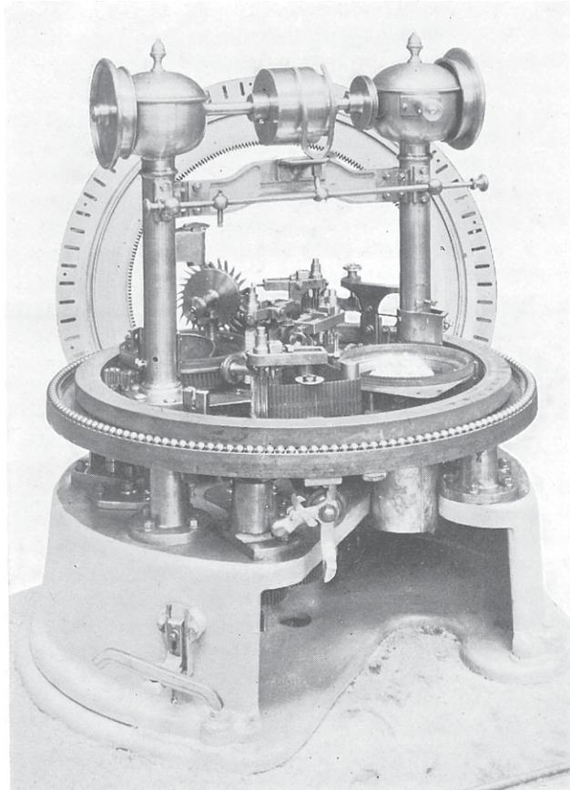
Fig. 96.—The Noble Horizontal Circular Comb
