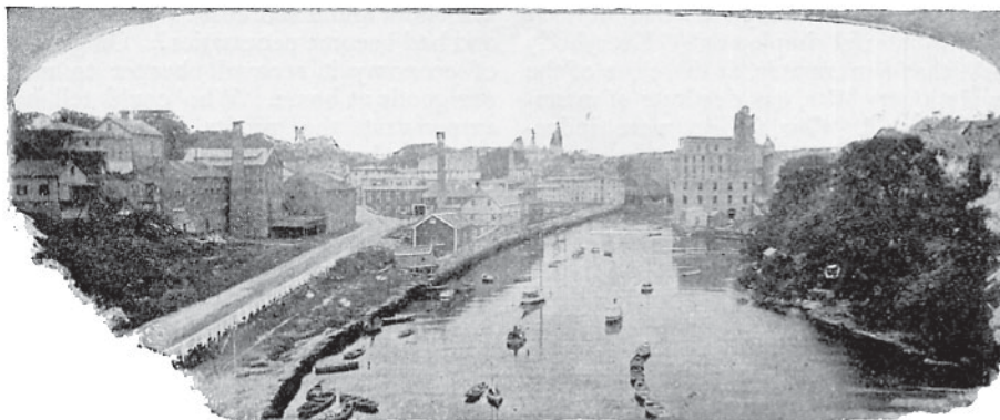
View of Pawtucket from the Division Street Bridge.
